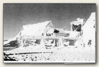
the Tip Top house. It had two stories at the time and we lived in the top story *(left)*. It had been "winterized" for winter use by a heating system, some indoor living improvements and insulation of blown in Vermiculite. The insulation didn't last long because the first wind over 100 mph blew it out again. AIRL had lived in it previously and got some of its shortcomings fixed. During the time we were on Mt. Washington, the Yankee Network only transmitted FM music. We had a
