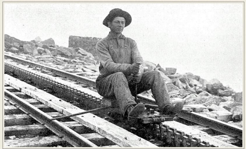
Pike's Peak - Similar, But Different: The Colorado cog railway was of a similar, but different design - both in the center cog rack, and the workers' "hand cars" to descend the line. The western boards were not as wide and ran outrigggers to the outside rails for stability. (1904) - Catskill Archive Collection /www.catskillarchive.com/rrextra/pikepe11.Html
