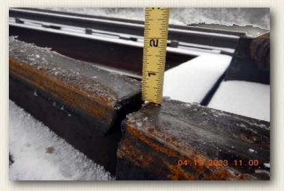
**Remedial Action 6:** Loose joint bar (jointed track). Located on the passing track north of the lower switch at Waumbec Station, east rail *(right)*. Gap measured 1-1/8 of an inch. Remedial Action: Yes Comment back to NHDOT
