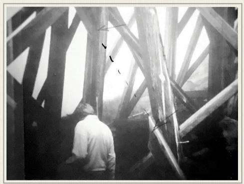
NH Bridge Design Breuau personnel inspect Bent 680 - finding diagonal bracing cut out, right side as indicated by dotted line on photo (May 1986) - NH Transportation Dept files
