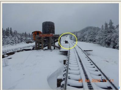
**Remedial Action 11:** Area of concern. Up passing loop, bent number 150, track curving to the left outside rail visually reverse elevation. Risk "low" owing to very low speed of the train at this location. Additionally, mast at side of track also leaning away from the structure. See photo 11a *(left)*. Note: As not regulated by FRA for further guidance only, reference CFR 49 relevant part 213.57. Investigate and report back to DOT.
