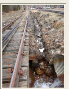
*Remedial Action 5:* Each drainage or other water carrying facility under or immediately adjacent to the roadbed shall be maintained and kept free of obstruction, to accommodate expected water flow for the concerned area. Multiple locations were found with either blocked culverts or
