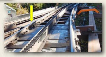
Cog Railway Track & Trestle Safety Standards. Section 3 Rail joints (d) "maintain the alignment of the abutting rail ends. Photographs attached *(right & previous page)* Correct and report back to DOT"
