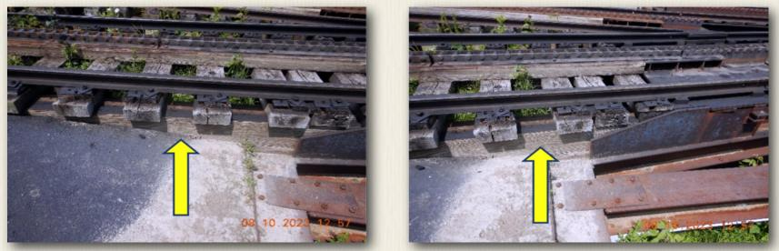
**Remedial Action 5:** There shall be at least four (4) non defective ties every twelve feet (12') of track. Rotted and or split ties visually identified at multiple locations *(below)*, spans 65/69/72/73 (#12) 142 (#2) 218/219/222/239/241/242/25/252/262 (#15) 384/385/395 (#6) 1023/1178/1179 (#5). Remedial Action: Yes Comment back to NHDOT (within 30 days of the inspection)
