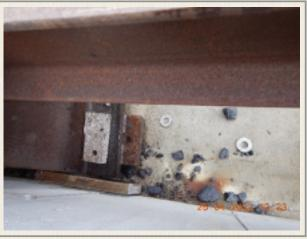
**Remedial Action 2:** Bents 70 through 150 located on the up passing loop at Waumbek Station, high number of base plates rotating outwards from under the rail base. Track shall be kept fastened by a system of components
