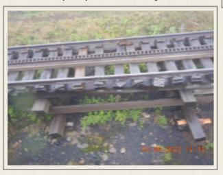
Action 1: Bridge between bents 8-20. I observed movement of the bridge decking which was attached to the track structure. Bearing plates two bolts located at the north end of the bridge, nuts had been removed, two bolts at the southerly end were missing, one was lying on the concrete base broken. Photos 1a through 1d at-
