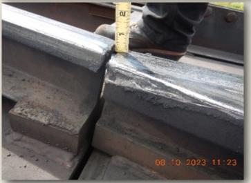
**Remedial Action 3:** Mt Washington Cog Railway Track & Trestle Safety Standards. Section 13 Inspection of Hydraulic Shuttle Switches (b). Mismatching of rack or running rail at any transition point shall not exceed 3/8 of one inch. Rail end mismatch on tread located between frog transition measured at + 3/8 of one inch upper Waumbec switch, main track *(left)*. Remedial Action: Yes Comment back to NHDOT (within 30 days of the inspection)
