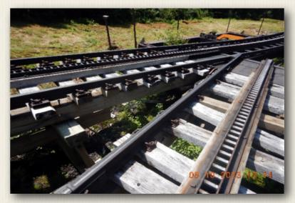
**Remedial Action 6:** There shall be no more than four and three quarter inches (4-3/4) between upmountain spool faces. Located at the base of the south (Waumbek) switch measured 4- 13/16 inches, rack has visual signs of movement *(below)*. Remedial Action: Yes Comment back to NHDOT (within 30 days of the inspection)
