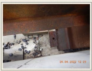
tached. *(left & right)* Note: As not regulated by FRA, for further guidance only, reference CFR 49 relevant part 237. Investigate and report back to DOT, missing anchor bolts
